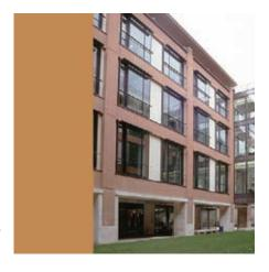
This Arup Associates building at **80 Cannon St.** / Bush Lane dates from 1972 - 6 and employs an exo-skelton which leaves a column-free interior. This stainless steel structure is said to be water filled as fire protection (suggesting
