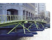
sliding connections to concealed concrete piles under the water. The central portion is hydraulically operated (assisted by counterweights) and opens to allow boats through. But there is a curiously neo-militaristic undertone — as if some romantic, war-weary 'band of brothers' was about to march over.
