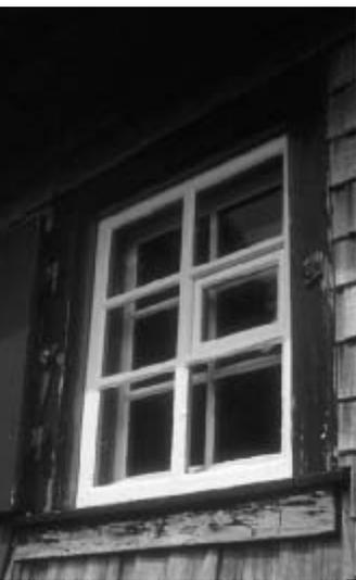
36. The hut's windows have two layers of glazing, both of which open for variable degrees of ventilation. Some windows—like this one to the dining area—also have an additional small opening light in the outer leaf.
