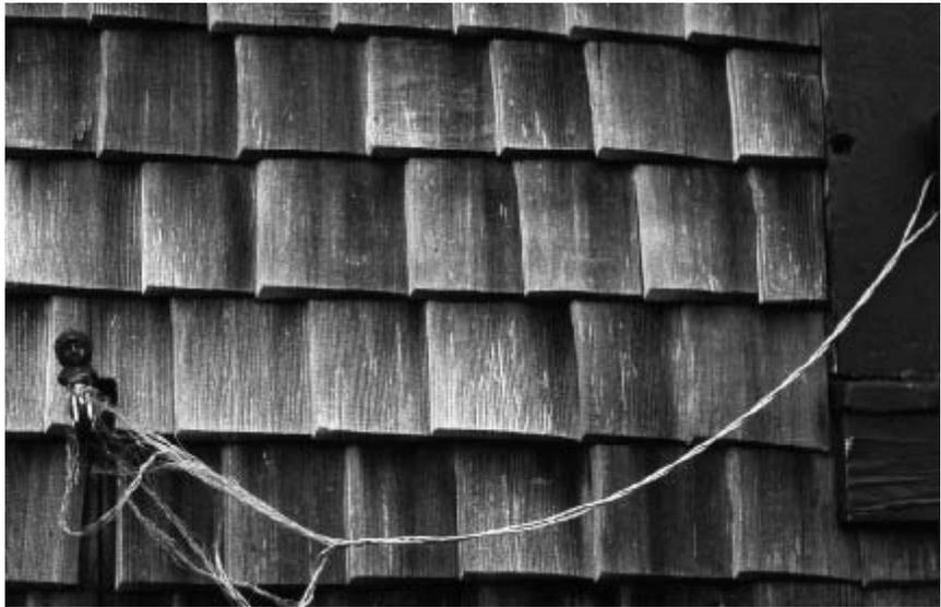
17. Externally, walls are clad with timber shingles in equal courses, lapped in two directions.
