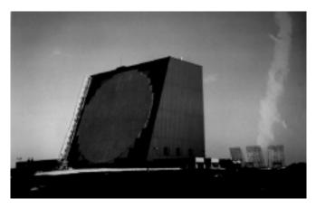
**Figure R37** Cobra Dane phased array reentry instrumentation radar (Raytheon Co. photo).
