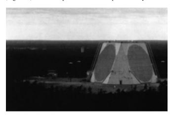
**Figure R60** Pave Paws missile-warning radar (from Brookner, 1988, Fig. 4.1, p. 280).
