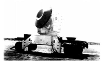
Figure R22 Nike Hercules monopulse fire control radar.
