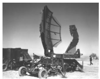
Figure A76 AN/TPS-43 stacked-beam reflector antenna.
