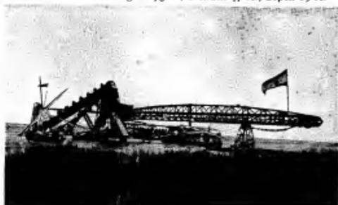
FIG. 6.—Light-draught dredger, with delivery apparatus working round an arc of  $210^{\circ}$ , by Hunter & English.
